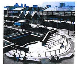
framing of central space
